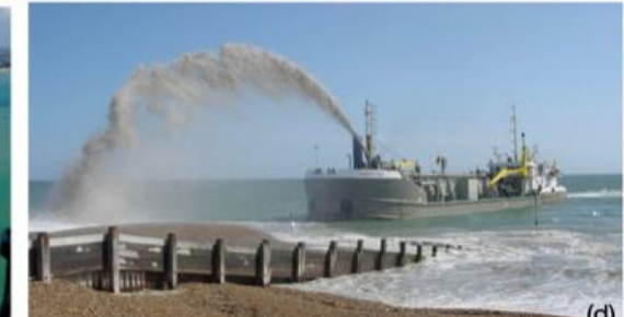
Hard protective structures for coastal management: (a) Seawall in Isle of Wight (Source: Oikos-team, 2007); (b) Groynes in Sitges, Catalonia, Spain (Source: Jordi Serra, 2007); (c) Detached breakwaters in Brazil (Source: UFPE); (d) Beach nourishment in Hayling Island, England (Source: ESCP); (e) Accommodation & Advance responses (IPCC, 2019)
